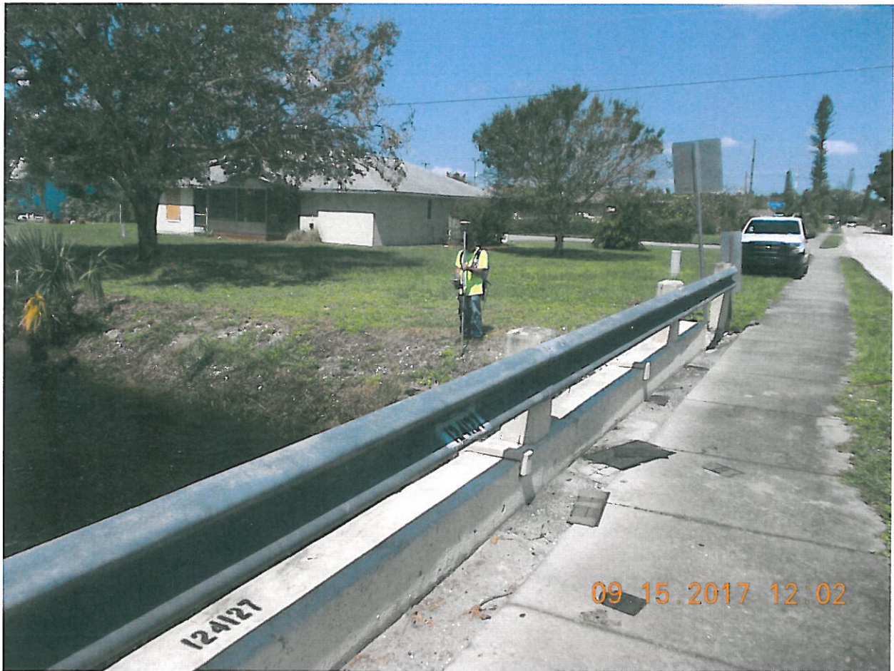
West side of bridge
