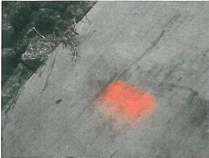
South side of weir
