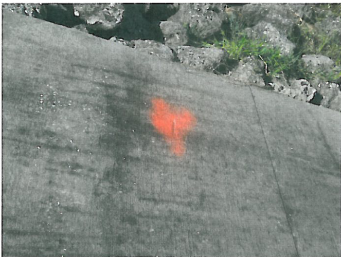
North side of weir
