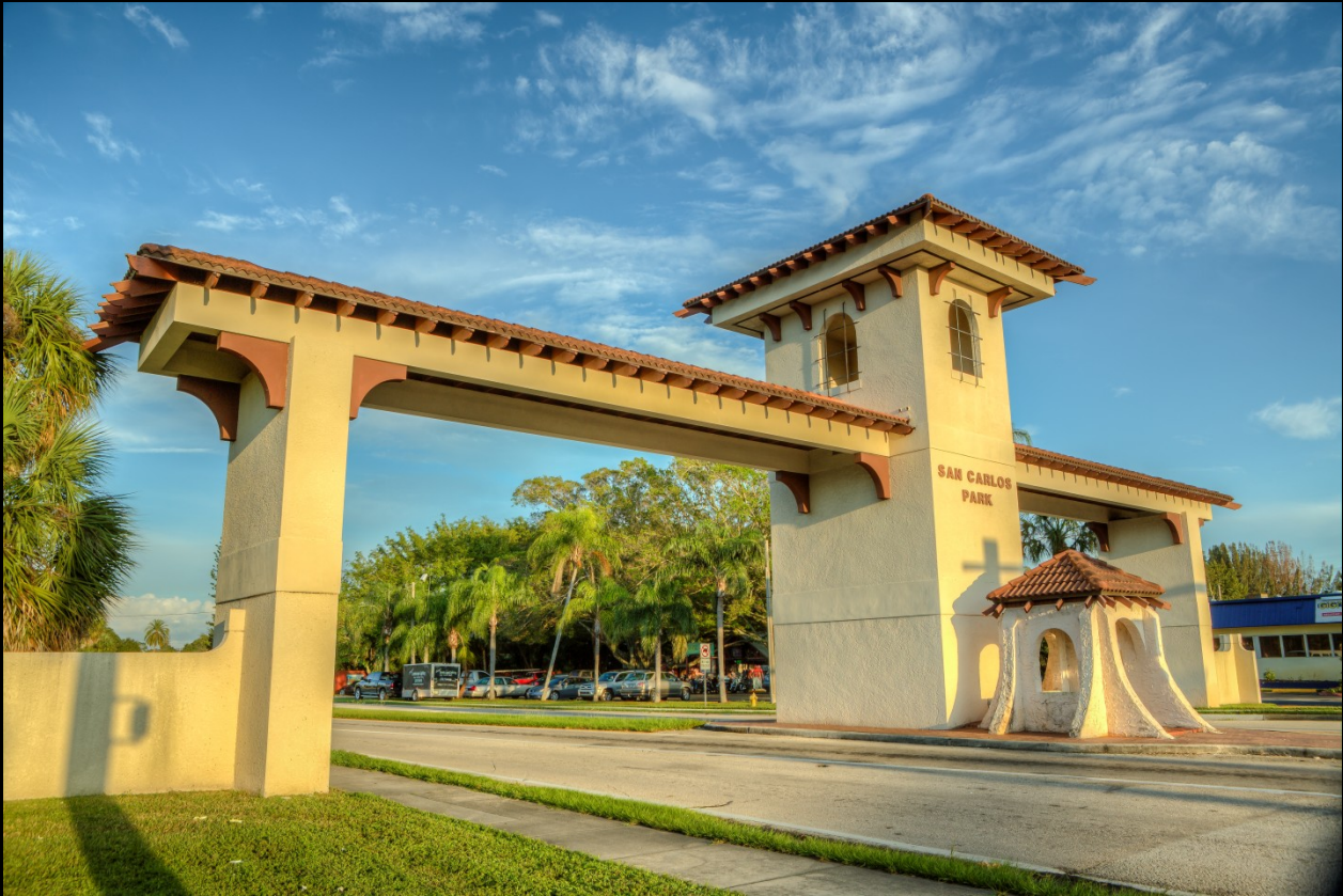
San Carlos Park Arch
