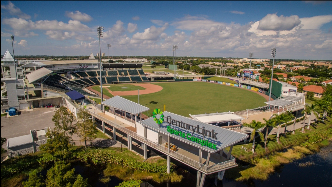
CenturyLink Sports Complex – Home to Hammond Stadium
