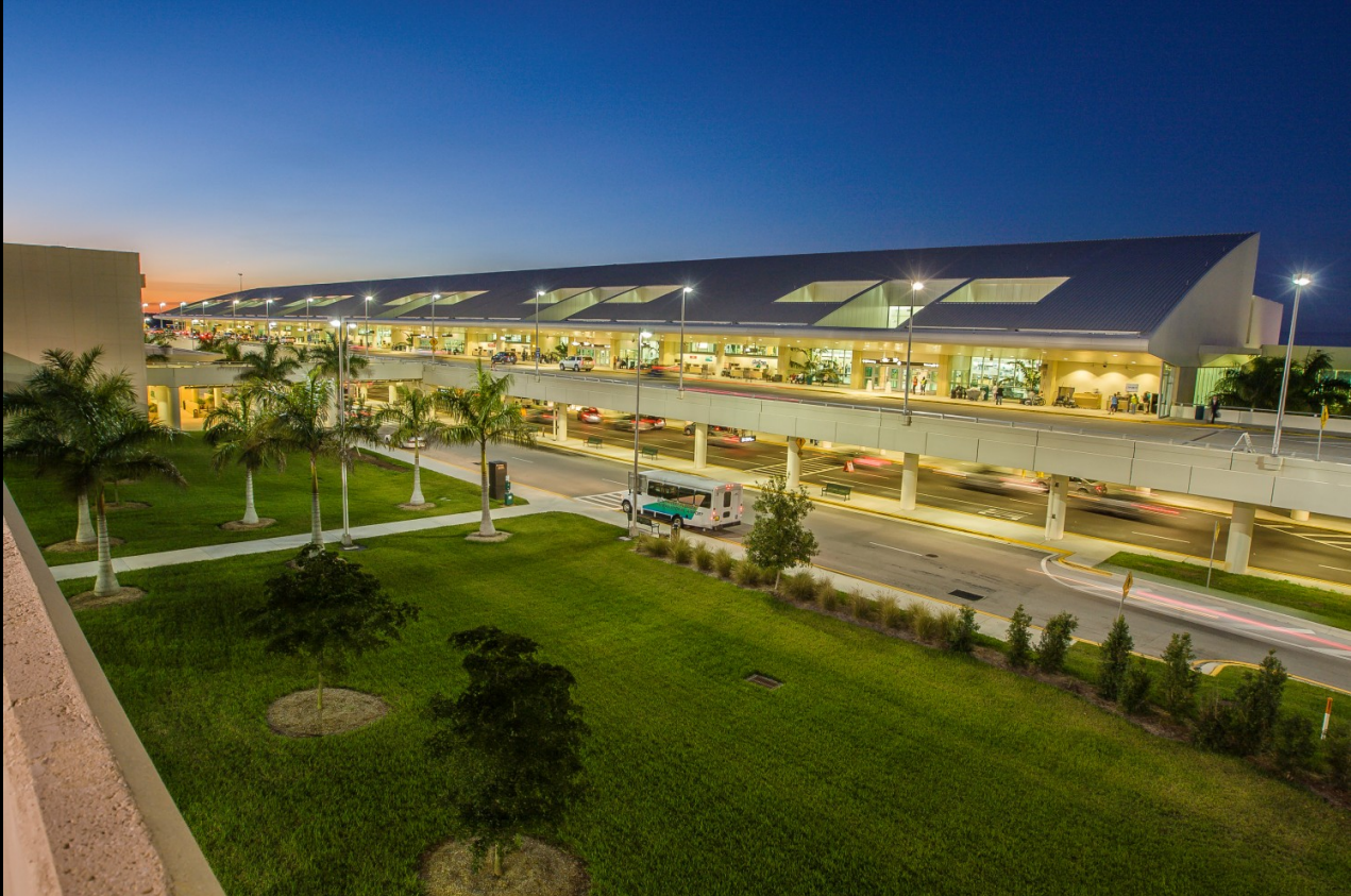
Southwest Florida International Airport – Midfield Terminal
